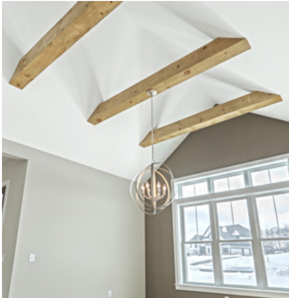
Rough Stained Collar Tie Beams
