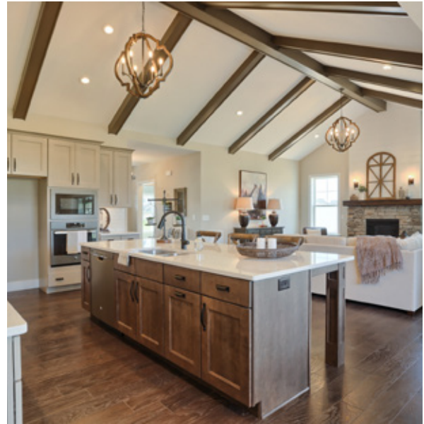
Painted Beams with 1/2" Reveal
