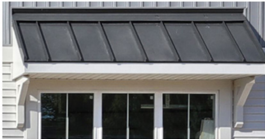
Pent Roof/Overhang Bracket
